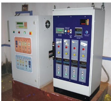
Bushlight India systems use high quality, standardised hardware, intuitive user interfaces and image based operation and maintenance manuals in local language to ensure systems are easy to use and maintain by both local operators and technical support agencies.
