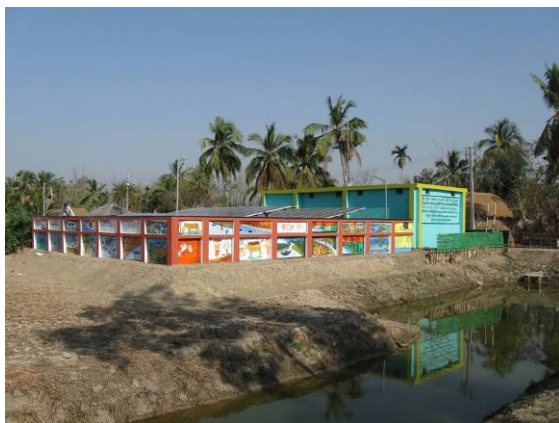
Figure 3: 9.63kWp Bushlight India solar PV system installed on Satjelia Island in the Sundarbans region of West Bengal, India. The system has a maximum design load of 23kWh/day.
